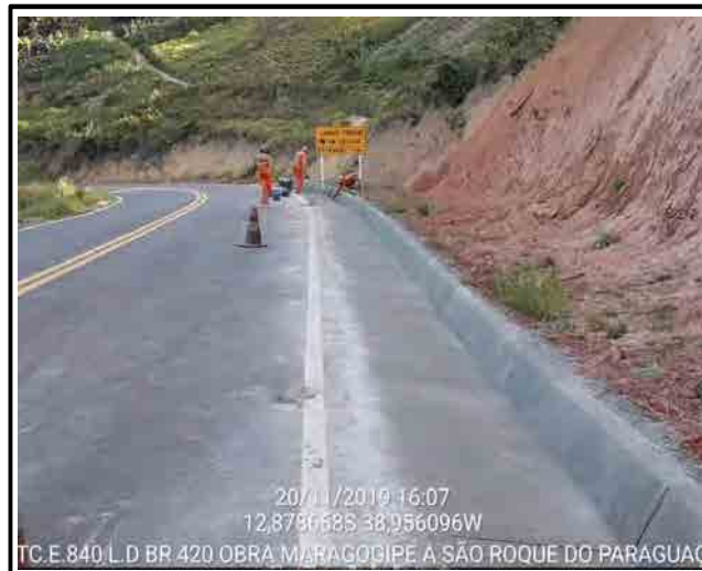
Corte E-830/850 LD Sarjeta executada
